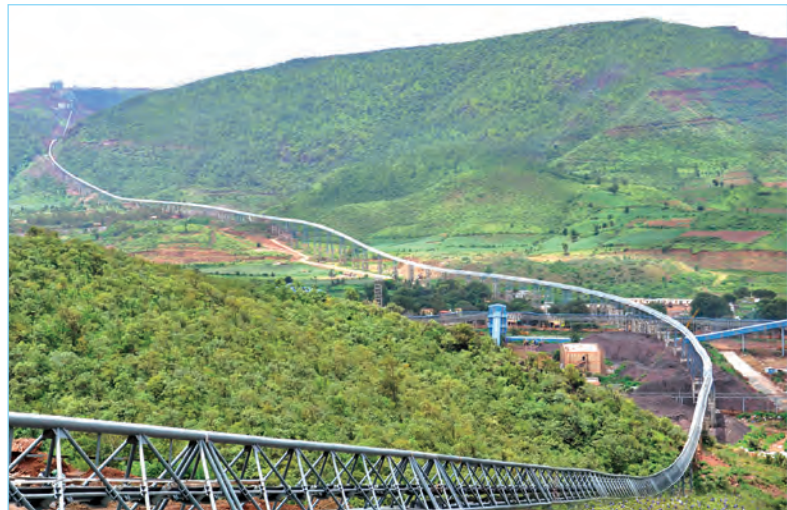
Panoramic view of the 5.2 km long single flight regenerative downhill conveyor belt at Kumaraswamy Iron Ore Mine, Donimalai, Karnataka
