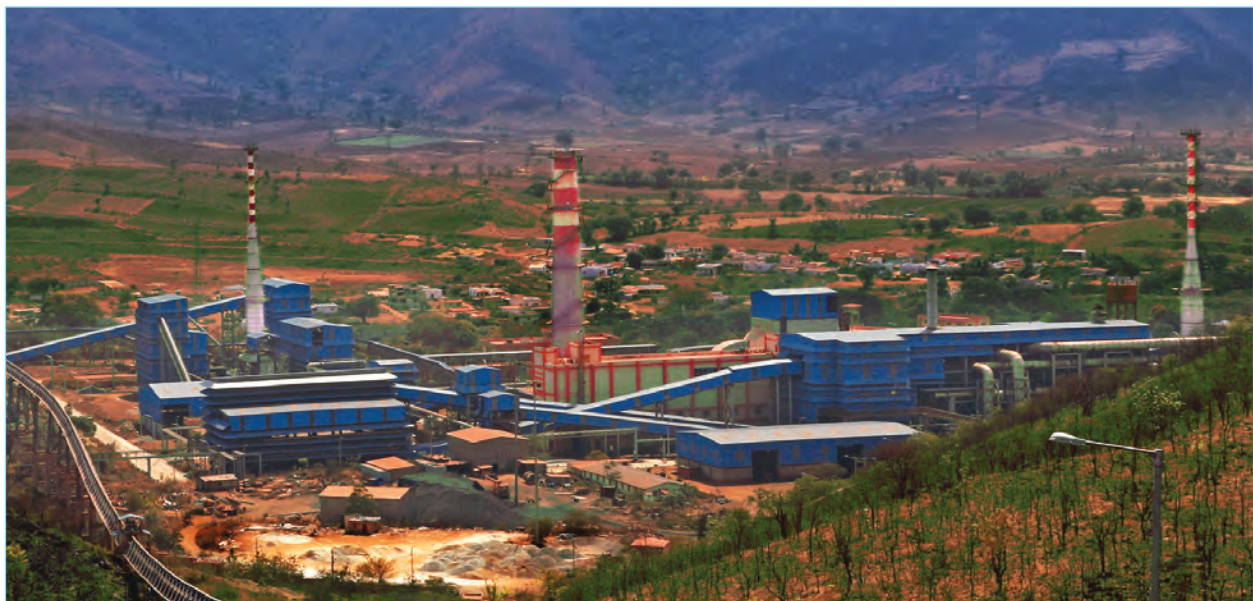
Panoramic view of Pellet Plant at Donimalai, Karnataka
