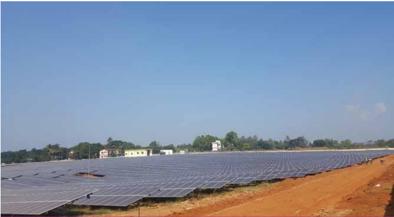
4 MW solar power plant for New Mangalore Port Trust (NMPT)
