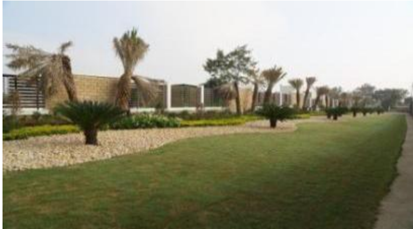
Landscape & Boundary wall
