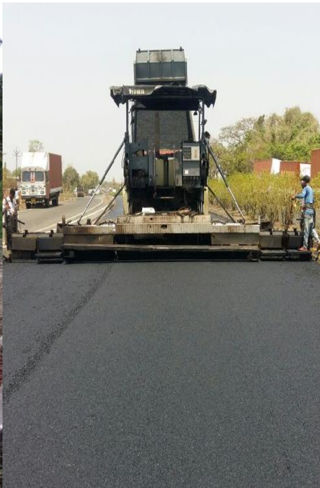
Major Maintenance Work at Nagpur- Kondhali Section
