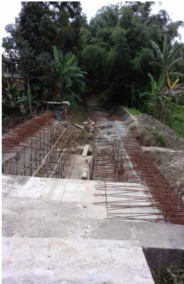
Vehicle Underpass at Moran Bypass (Assam)
