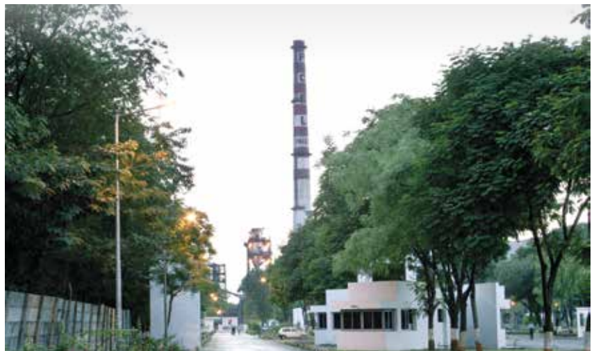
Palej Plant , Gujarat
