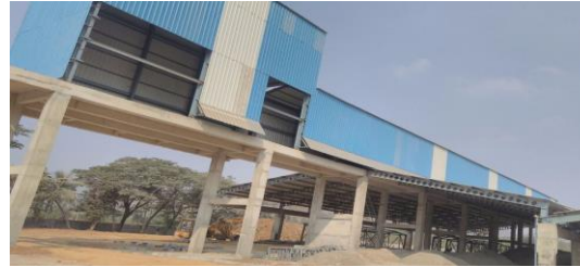
Raw Material storage facilities
