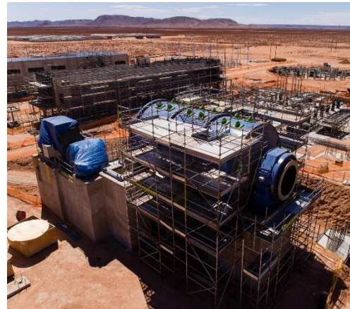
Erection of Ball Mill Shells, Bearing Housing & Motor
