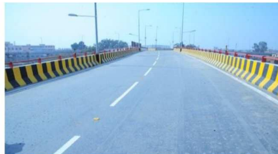
Construction of 2 lanes at Sonapat
