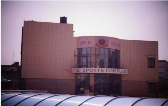
Police & Residential Quarters at Kandli, New Delhi
