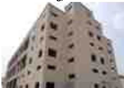
Multi-product/specialty chemicals facility Vizag, India
