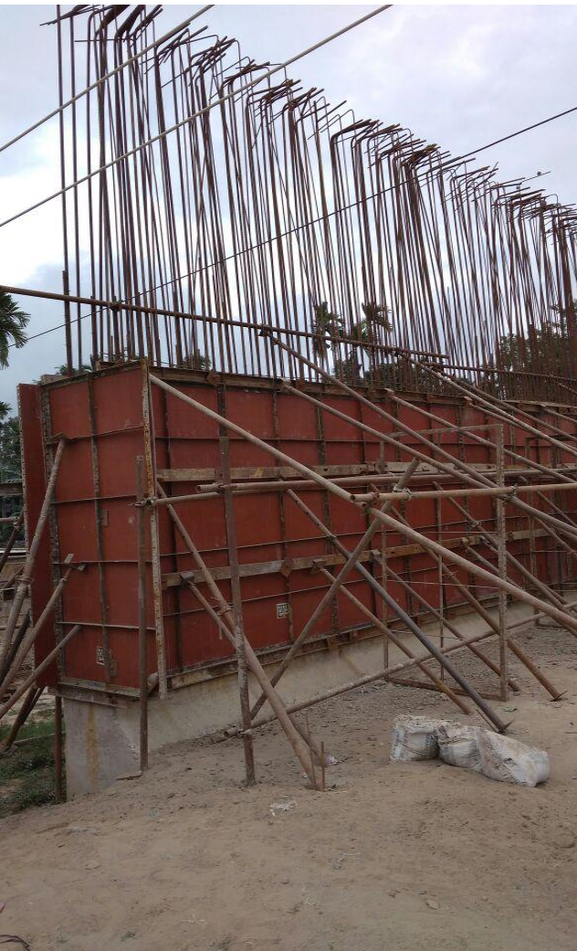
Vehicle Underpass at Moran Bypass of NH-37
