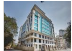
The Byke Suraj Plaza, Thane
