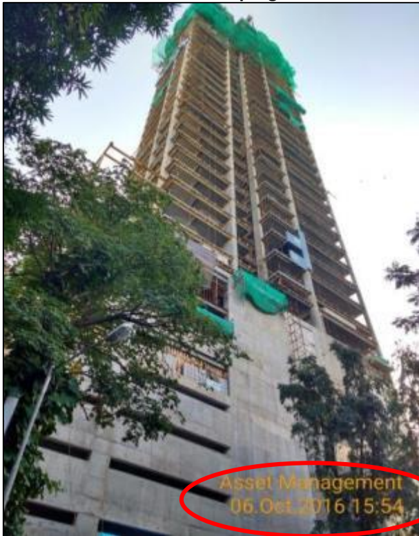
Oct'16 – RCC work in progress
