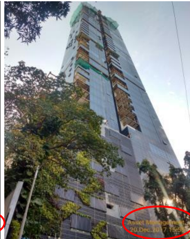
Dec'17 – façade work nearing completion
