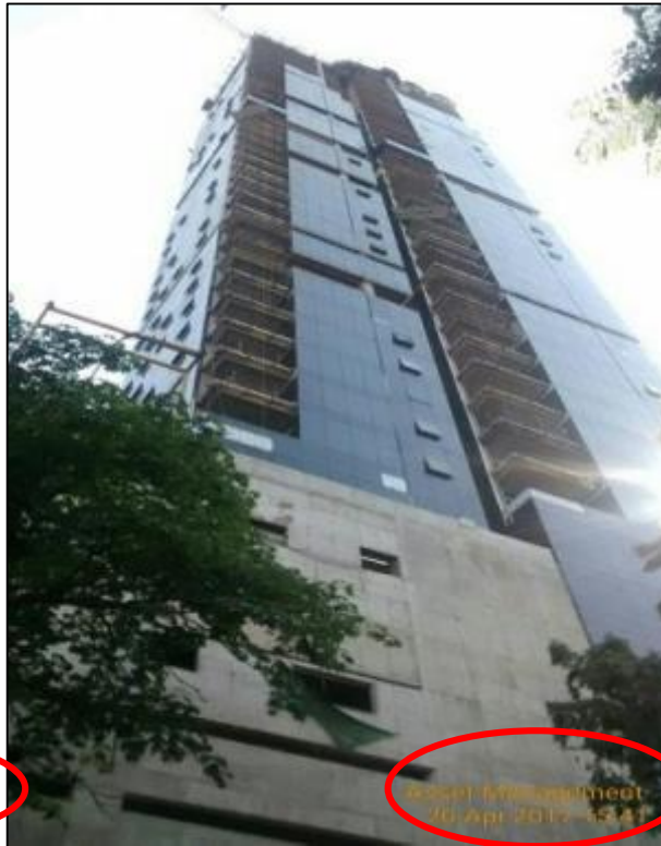
Apr'17 – façade work in progress
