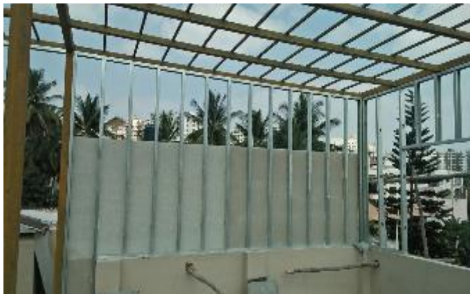
V-Infill wall partition at Residential project, Bannerghatta, Bangalore
