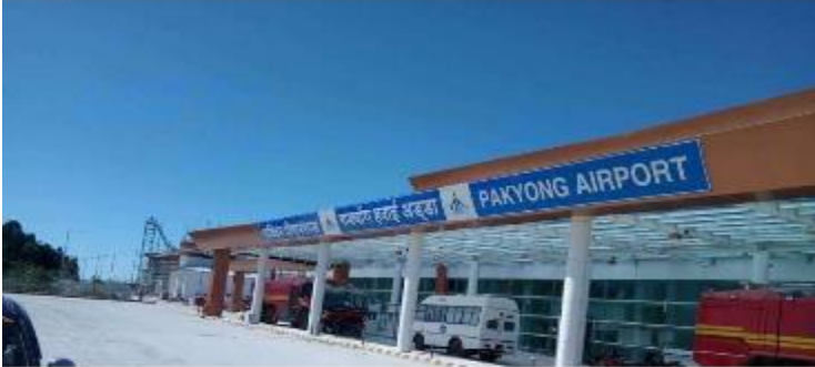
Pakyong Airport - Construction of Terminal Building Partitions
