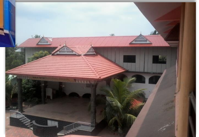
Roof Top Extension - (V-Panel )
