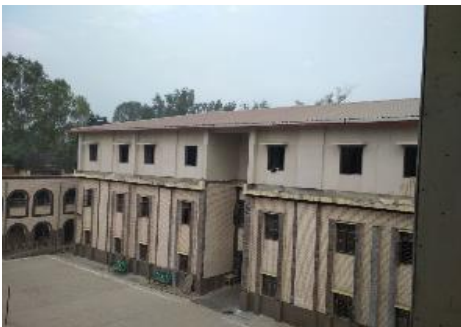
Sarvodya Vidyalaya School Project Partitions
