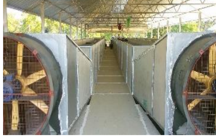
Moran Tea Factory Mezzanine / Partitions
