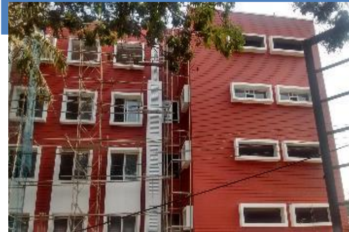
NATIONAL PUBLIC SCHOOL External cladding
