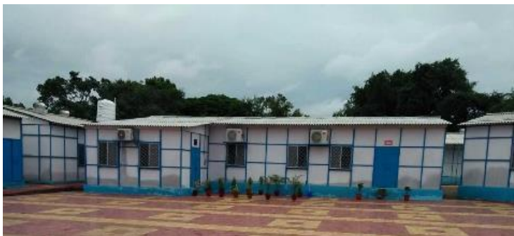
MES office Partition/ false ceiling
