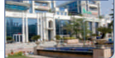
Post construction services
