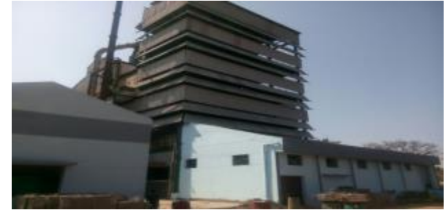
Unit 3 - New Reactive Dyes Plant
