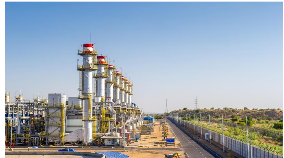
Mangala Processing Terminal
