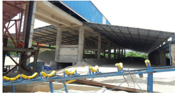
Raw Material storage facilities
