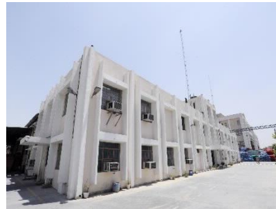
RFL I & II- Bahadurgarh
