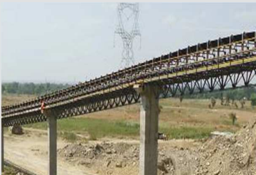
Overland Belt Conveyor
