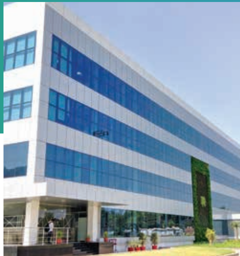
General Injectable Plant at Karkhadi
