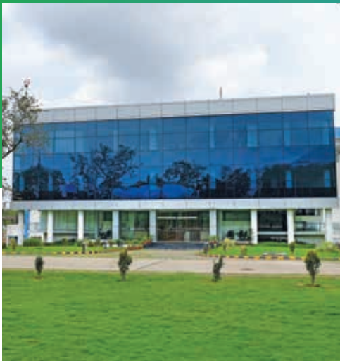
Oncology Plant at Panelav
