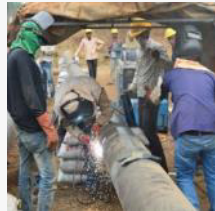
Thumbli Water Pipeline– Cairn Energy India – Rajasthan
