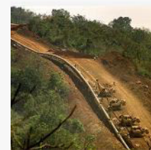
Panvel Dabhol Pipeline Project–Gail Ltd - Maharashtra
