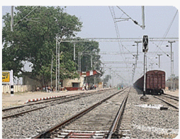
Mansi-Madhepura Electrification (Bihar)
