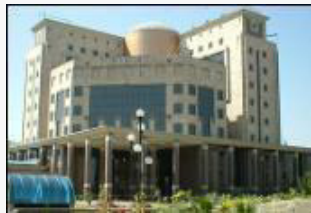
Power Grid Corpn., Gurgaon
