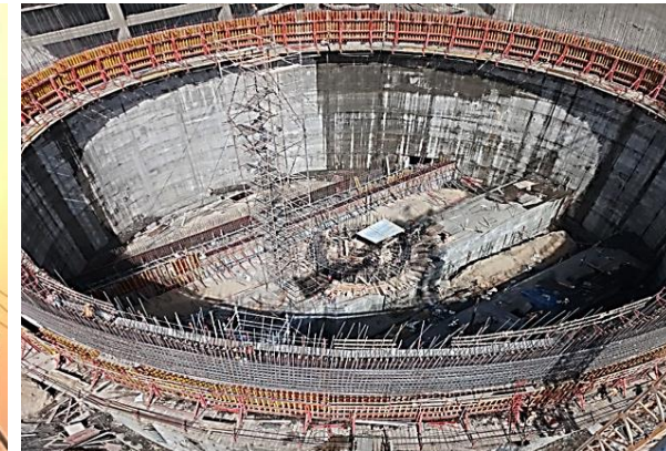
Construction of 55mt dia. Clinker Silo using Jump Formwork
