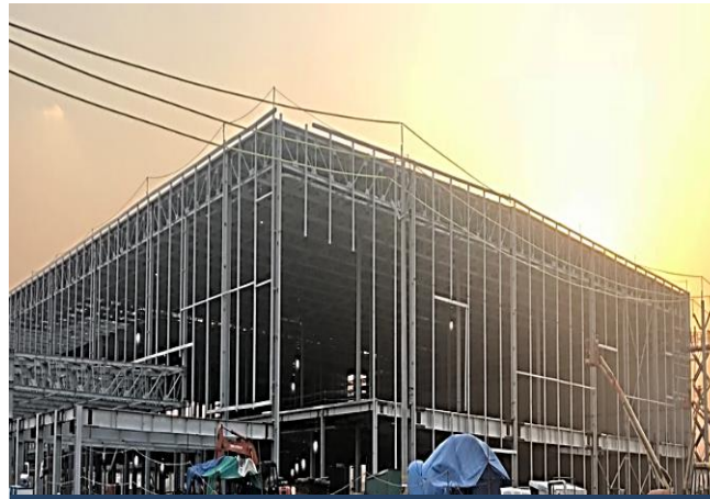
Structural steel works - Paint shop
