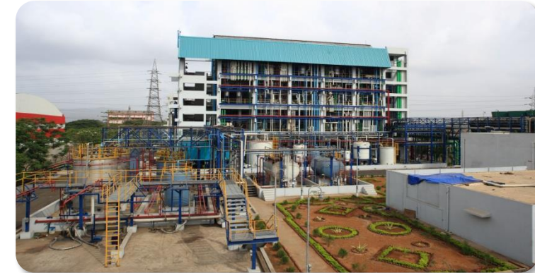
Agro Chemical Facility - Taloja
