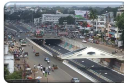
Grade Separator, Pune
