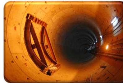
DMRC CC-24 Tunnel
