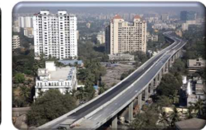
Flyover at Panjarapole, Mumbai
