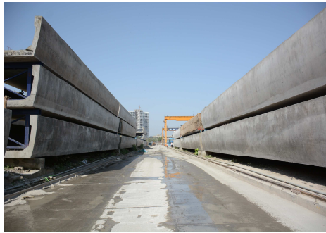
Bandra Casting Yard MML-07
