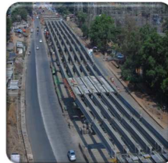
Mahape Flyover, Mumbai
