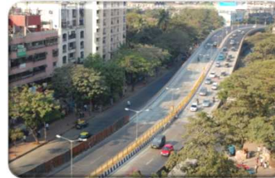
Flyover at Hindmata
