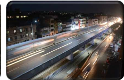
Flyover at Dhanakwadi
