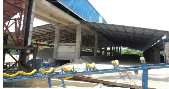
Raw Material storage facilities
