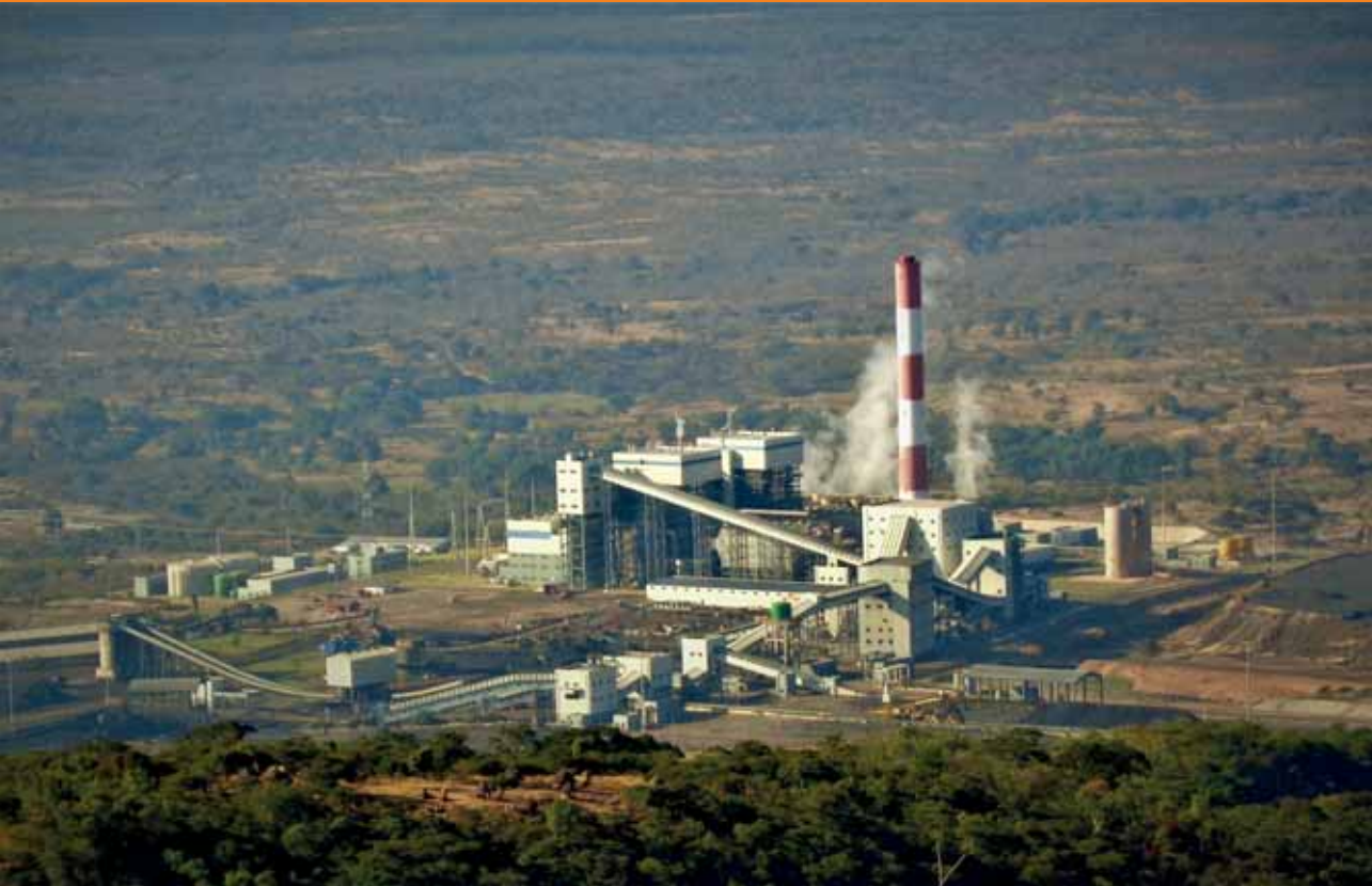
Maamba Collieries Ltd. Power Plant, Zambia
