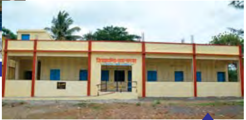
Salvad School : New Building
