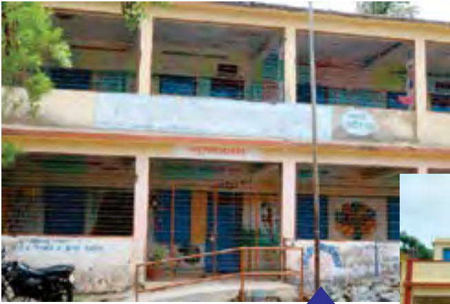
Salvad School : Old Building
