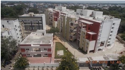
Construction of 92 flats at Bhopal
