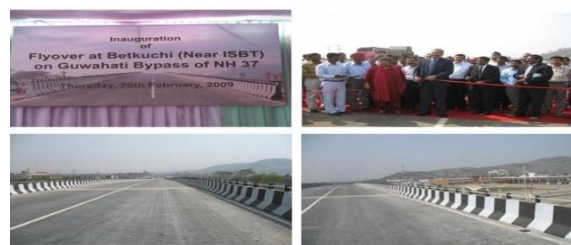
Construction of flyover in Guwahati
