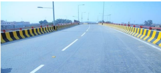
Construction of 2 lanes at Sonapat, Delhi
