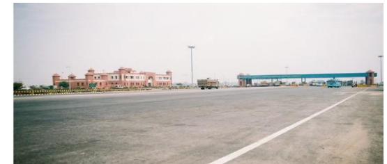
Toll Plaza construction at Delhi -Agra, NH-2
