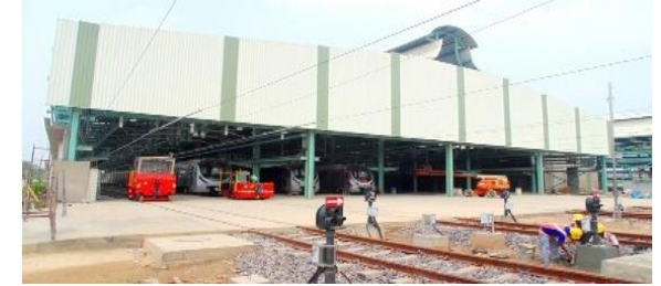
2 lane ROB at Sonapat-Purkhas Moi Road
