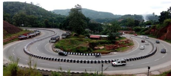
Widening and strengthening from 2 lane to 4 lane at Guwahati, Assam
