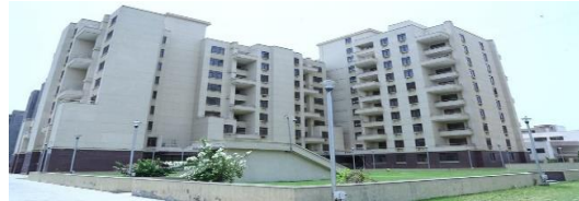
Residential construction at Dwarka, New Delhi
