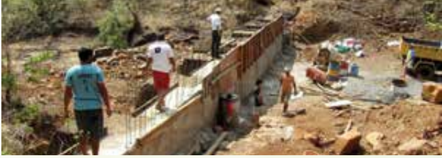
Permanent check dam structure at Sakhar village in Khed, Ratnagiri
