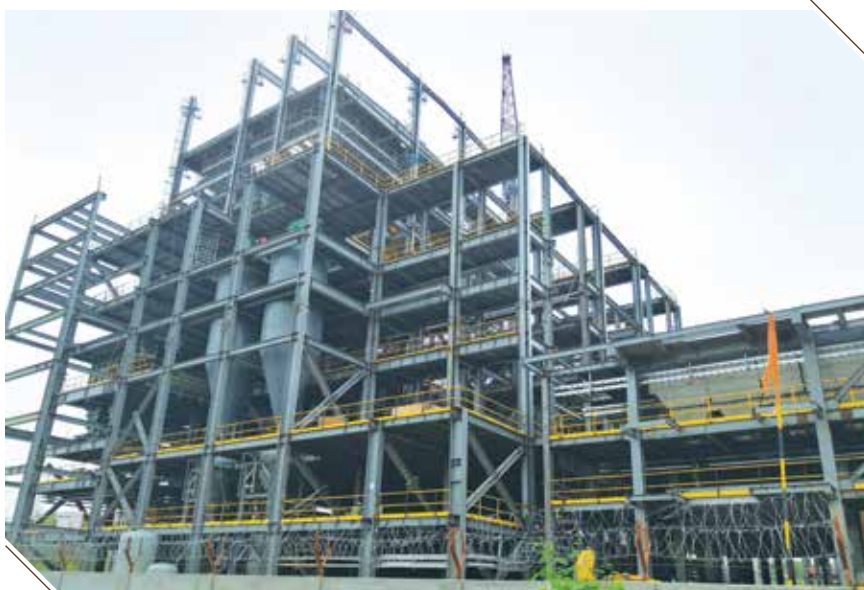
Fumer construction site - a step towards environment friendly technology
