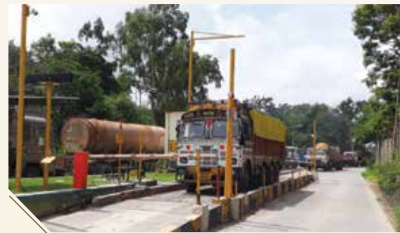
Technology upgradation: Man-less weigh bridge
