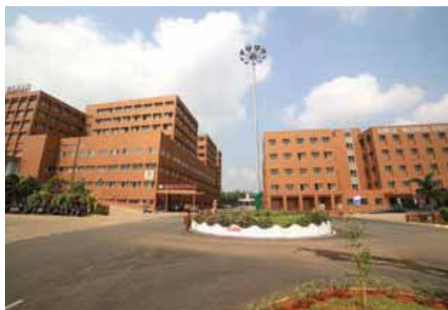
VRF, Packaged and Ducted system installations for Gitam University, Visakhapatnam
