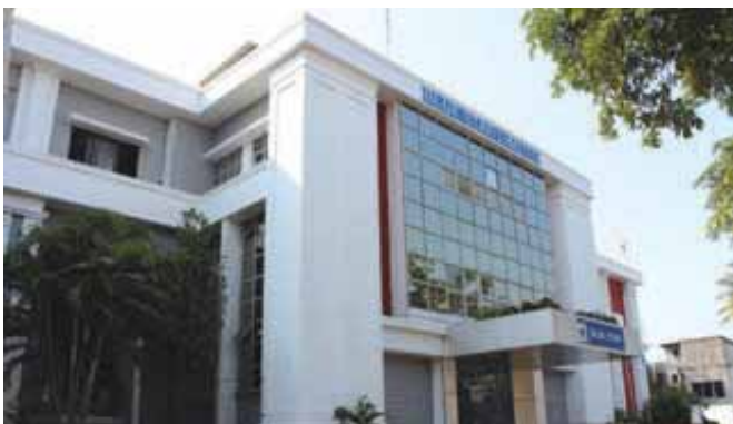
Blue Star's manufacturing facility at Dadra
