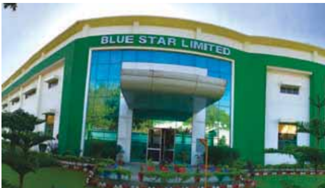
Blue Star's manufacturing facility at Himachal Pradesh
