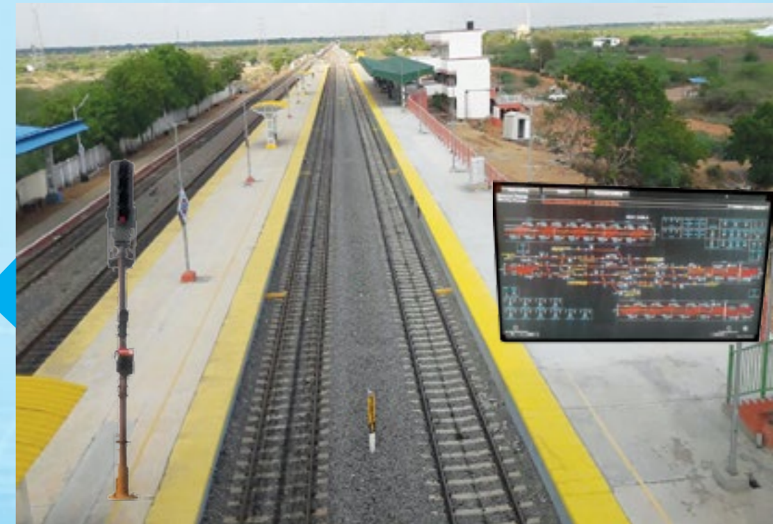
Thanjavur Railway Station and The Signalling Control of DFCC
