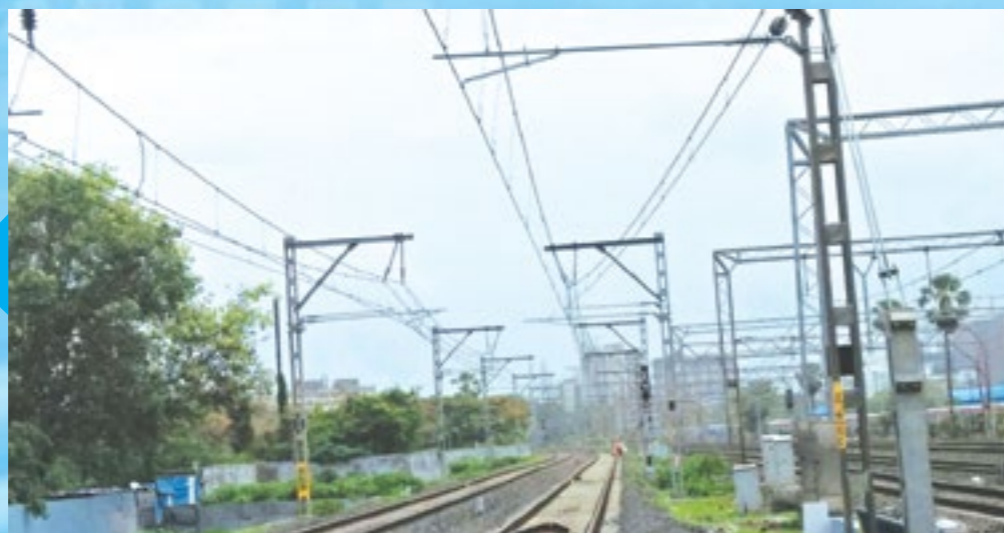
OHE Job on the Additional Lines between Andheri and Goregaon
