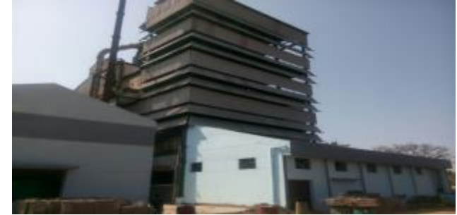
Unit 3 - New Reactive Dyes Plant
