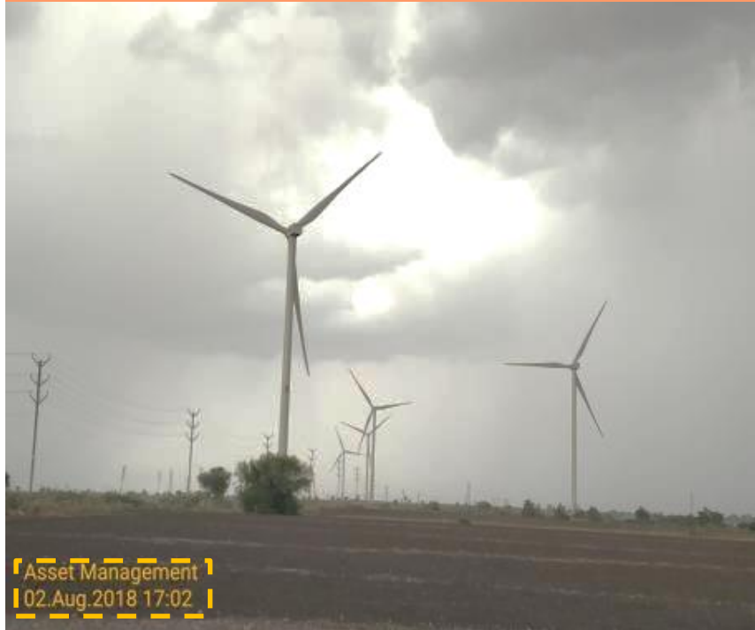
Operating wind turbines along with 33 kV lines
