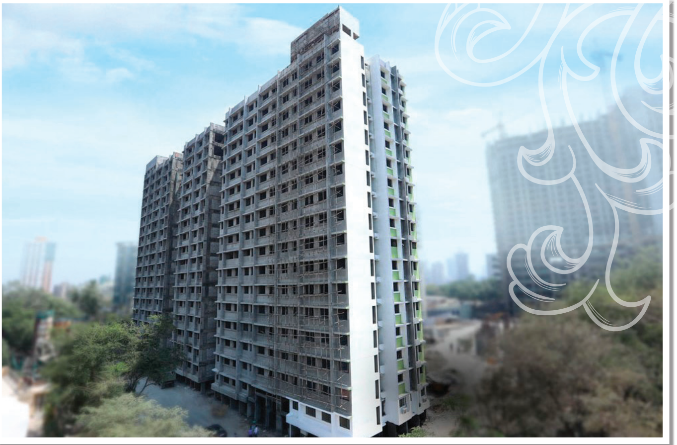
(Original Construction Project Photo)
