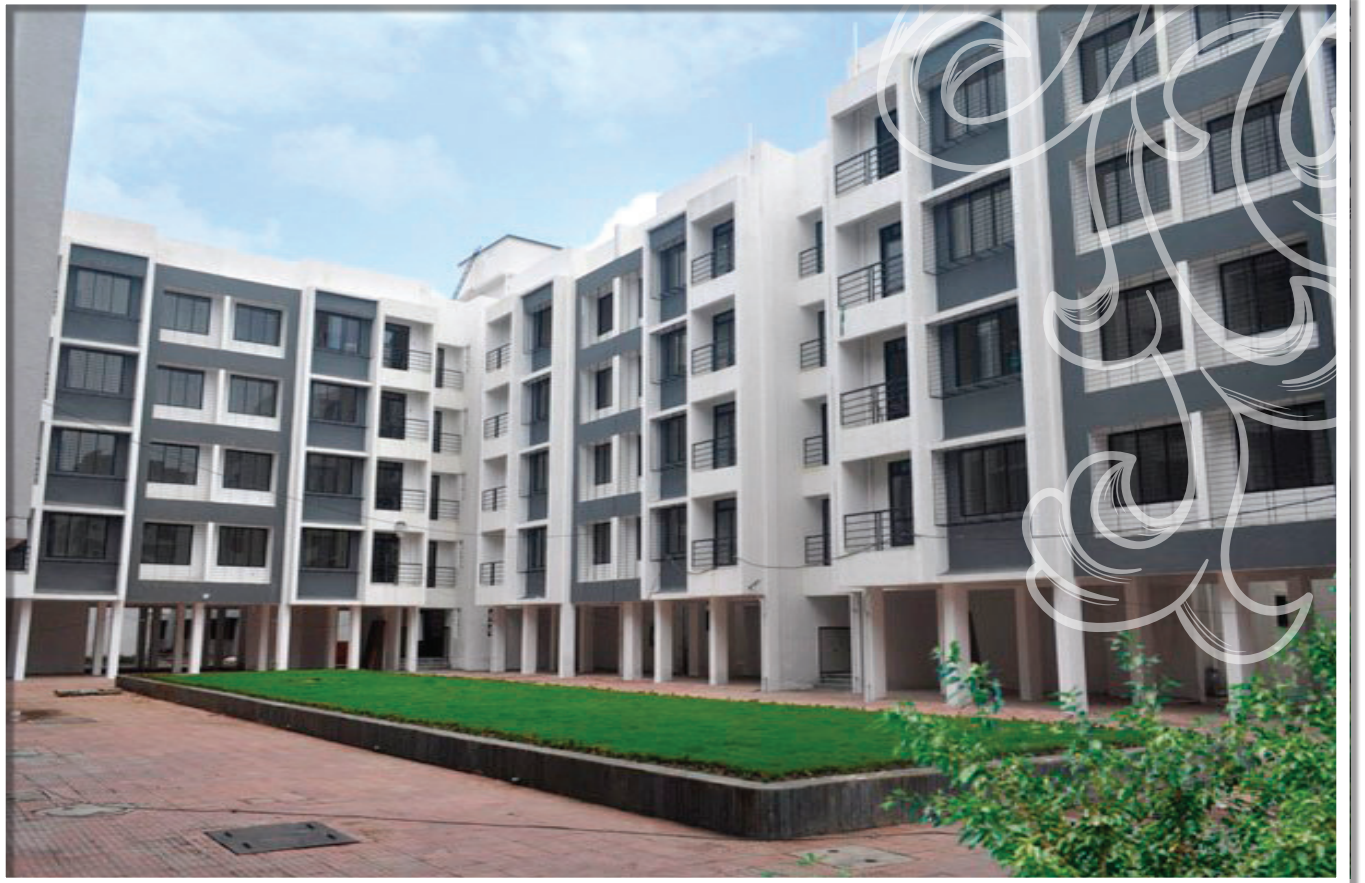
(Original Construction Project Photo)
