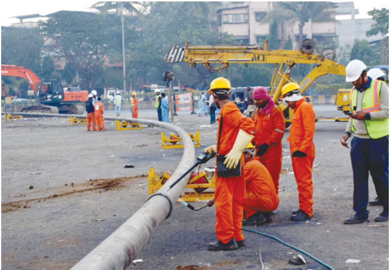
◆ Laying of pipeline at Durgadi creek
