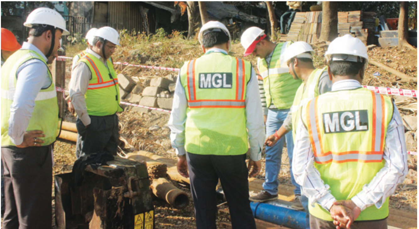
● Laying of pipeline at Durgadi Creek
