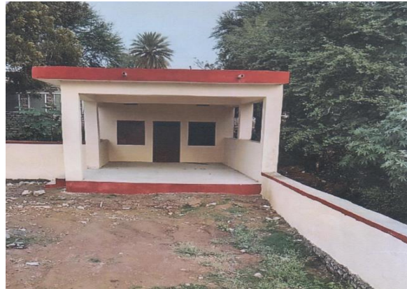
Community Hall Construction at Nimbahera
