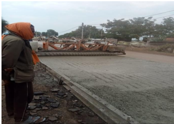
Construction of Village Road at Panna
