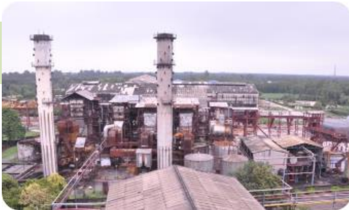
Sugar plant overview
