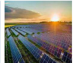
Solar Mounting Structures
