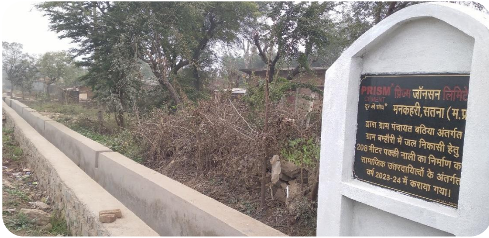
Construction of Drain at Bamhauri
