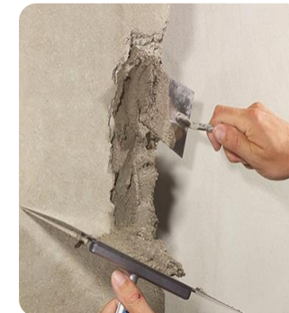
Concrete Repair, Anchors & Grouts
